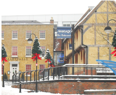
View from High Street
